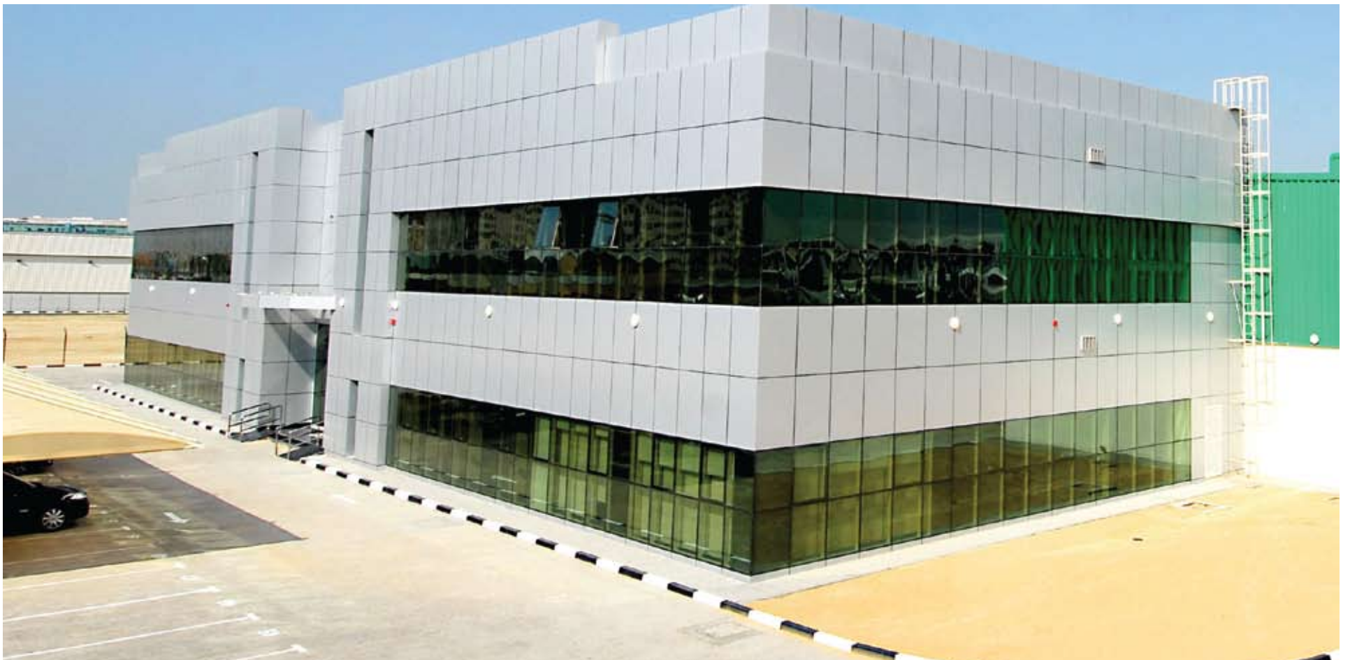
DTTC facility in Jafza South
