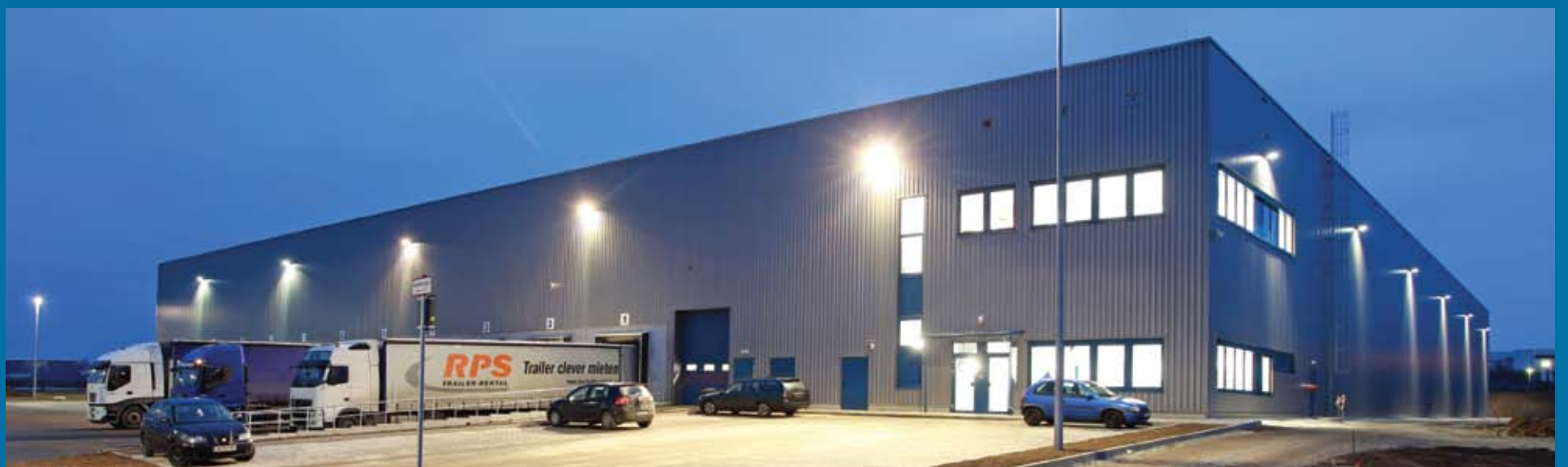
Gazeley recently delivered 10,000 m 2 state-of-the-art warehouse to Axthelm-Zufall at Nohra in Germany
